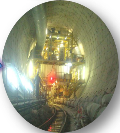
River Diversion / Bypass
